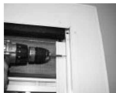
FIG 10: Re-attach channel
