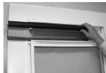
FIG 6: Rubber screen connector
