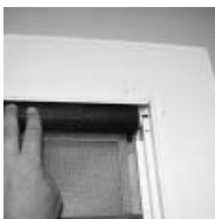
FIG 9: Insert right side of tube
