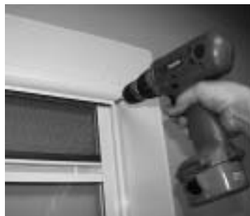
FIG 1: Head cover screw removal
