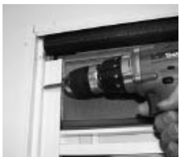
FIG 3: Channel screw removal
