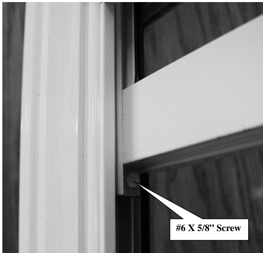
Picture taken from outside of door
