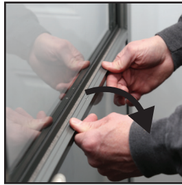
c. Rotate interlock extrusion towards you to disconnect.
