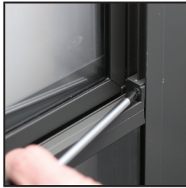
b. Remove (2) interlock anchors and (2) screws.
